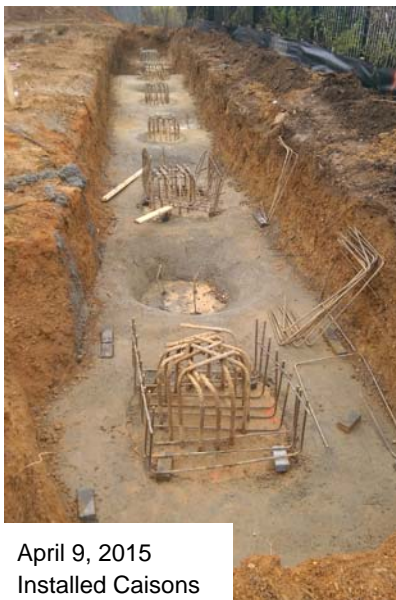
April 9, 2015 Installed Footings and Piers
