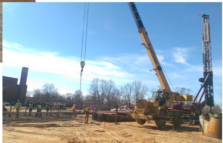
March 12, 2015 – Preparing to lift and install rebar cage for the caissons.
