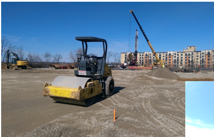
March 18, 2015 – Fill and grading building pad area, followed by soil compaction.
