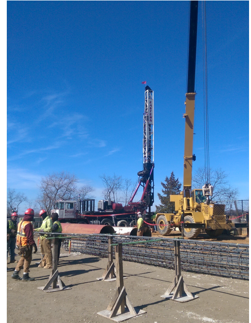
March 12, 2015 – Drilling caissons and building caisson rebar cages.
