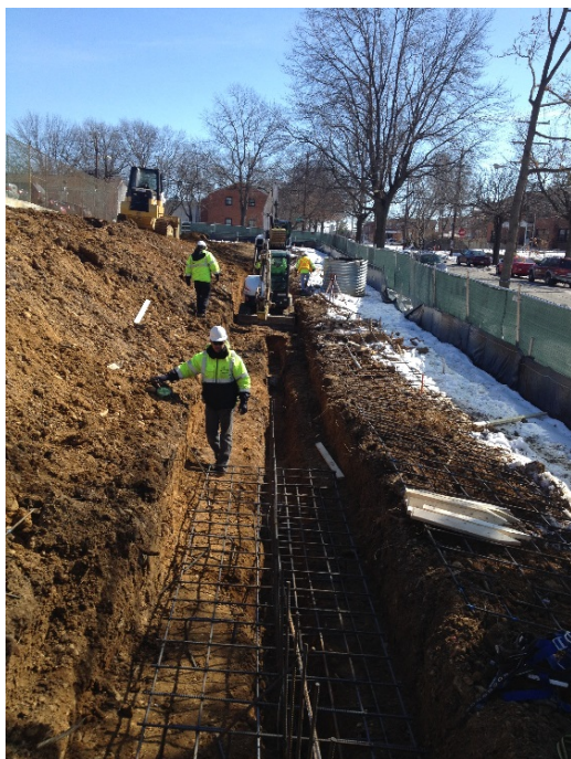
February 25, 2015 – preparing to pour concrete for the retaining wall
