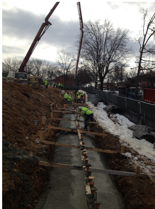
February 27, 2015 – first concrete pour for the retaining wall
