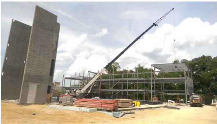
May 28, 2015 Steel Installation and Stair and Elevator Shaft
